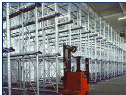
Drive-in Drive-through racking
